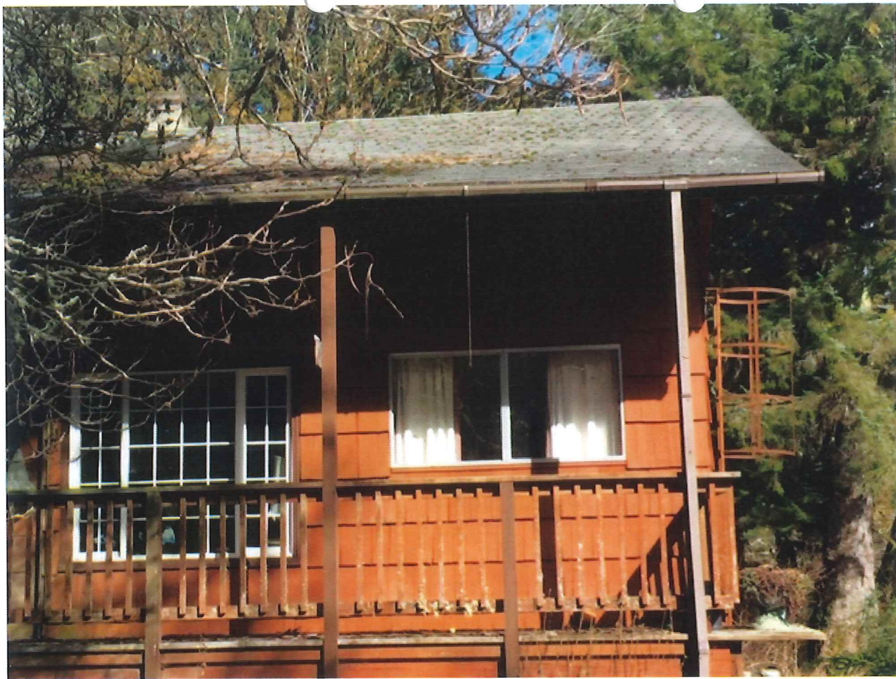
picture, exterior of dwelling
